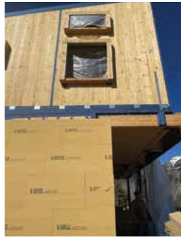
Credits Love | Schack Architecture - left: CLT structure w/ Guttex insulation, right: strawbale insulation
