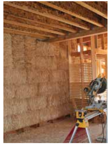
Credits Love | Schack Architecture - left: CLT structure w/ Guttex insulation, right: strawbale insulation
