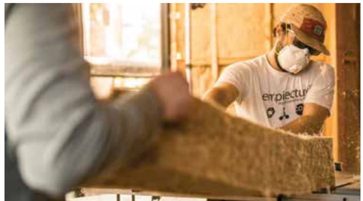
Credit Hempitecture - hemp batt insulation
